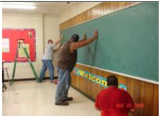
Maintenance preparing to install new marker board for JHS
